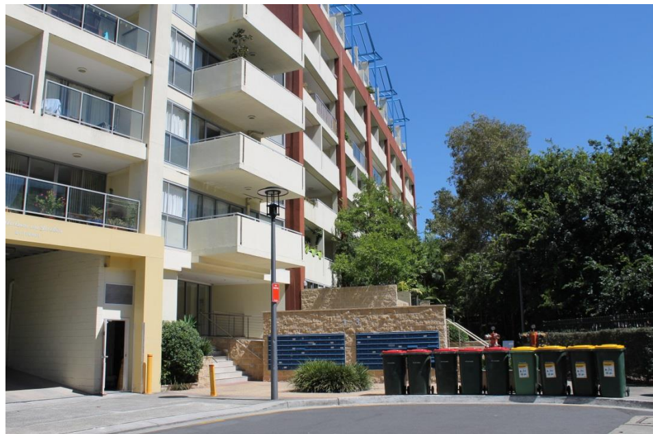
Figure 14 – Residential flat buildings located to the west and north-west of the site
