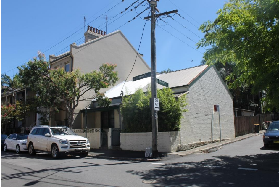
Figure 11 – Terrace housing to the east at the corner of David and Junction Streets
