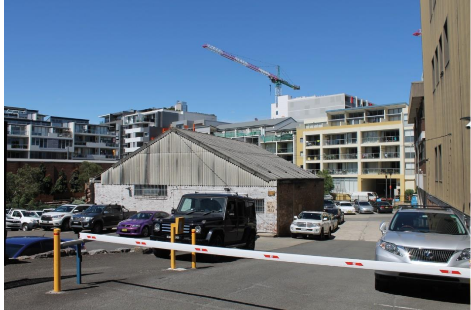
Figure 5 – Southern portion of the site as viewed from Junction Street
