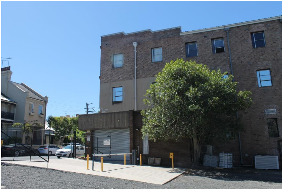
Figure 7 – Existing commercial building within the centre of the site fronting Junction Street
